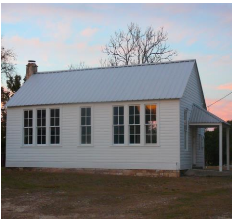
NEW PAINT INSIDE AND OUTSIDE AT RHEINGOLD SCHOOL-Looks great!
